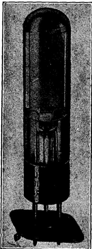
FIG. 8.—The "Burgess" selenium type light sensitive cell.
